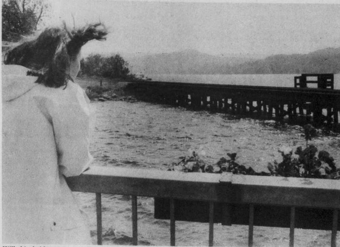
Will this bridge stay or will it be demolished?
